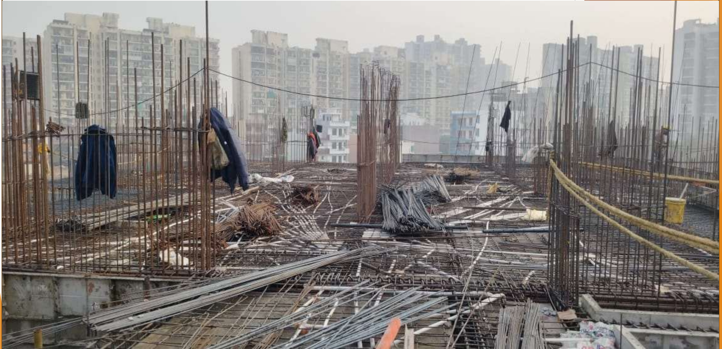
Tower 1B 4 th floor pour -1(Part -B reinforcement wip)
