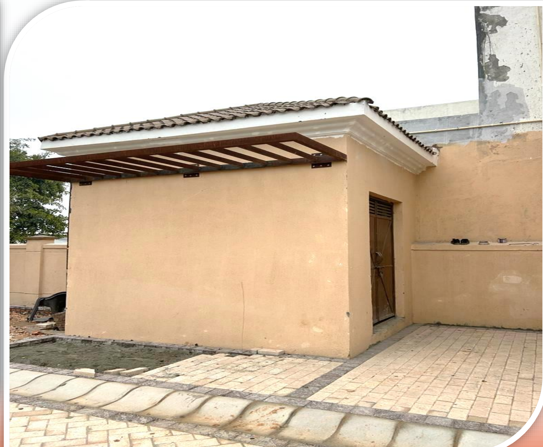
Meter room completed
