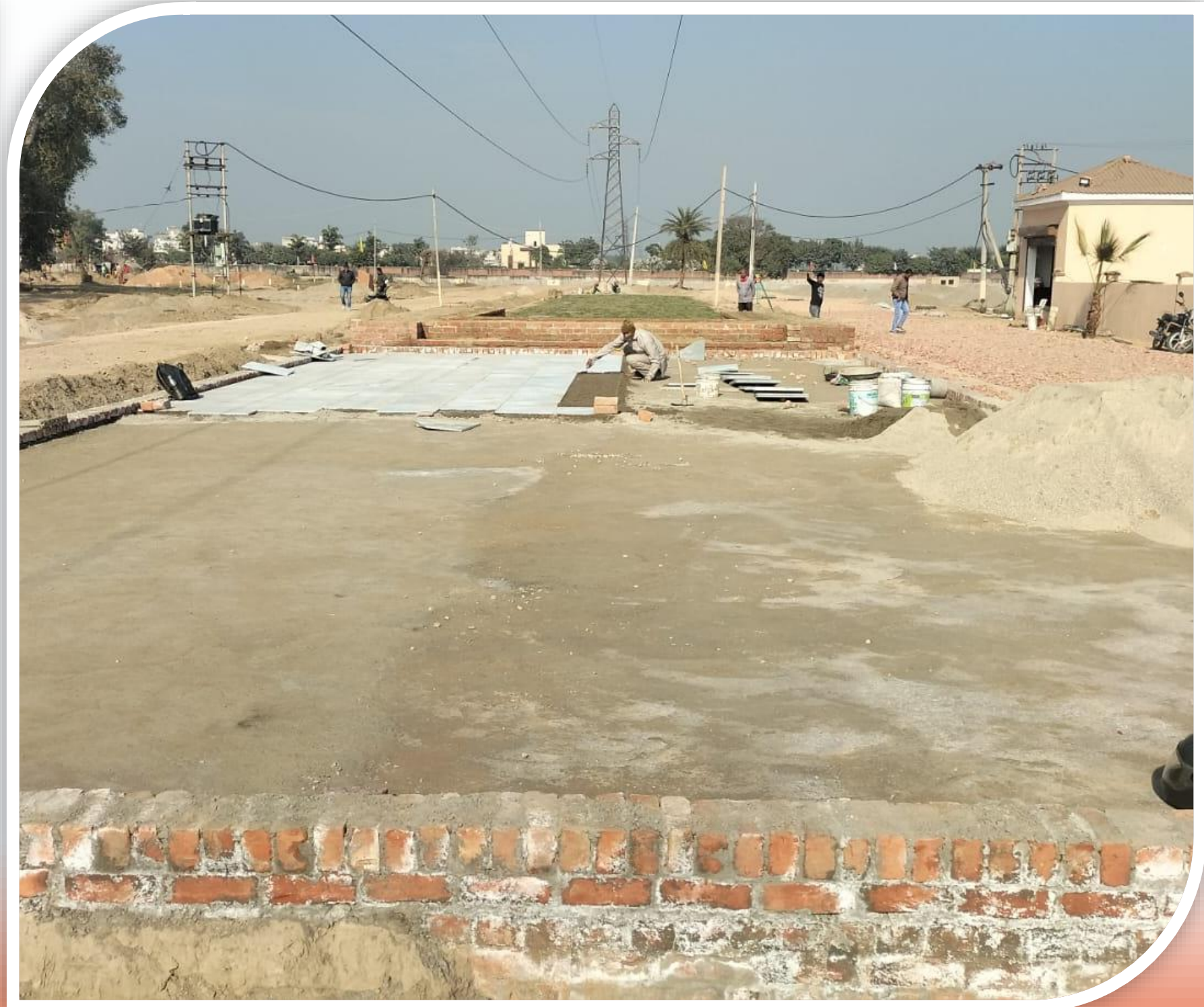
SKATING & GYM area civil work completed
