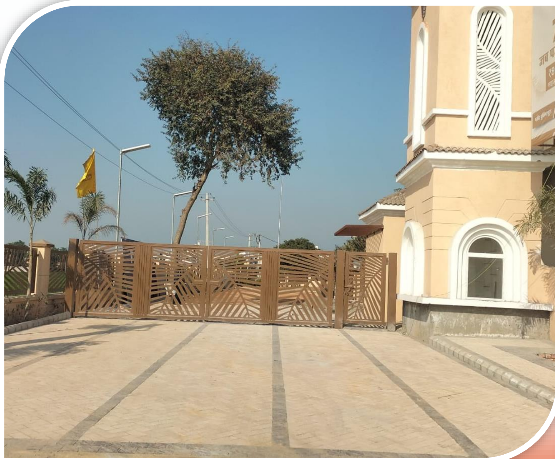
Entrance Gate Installed
