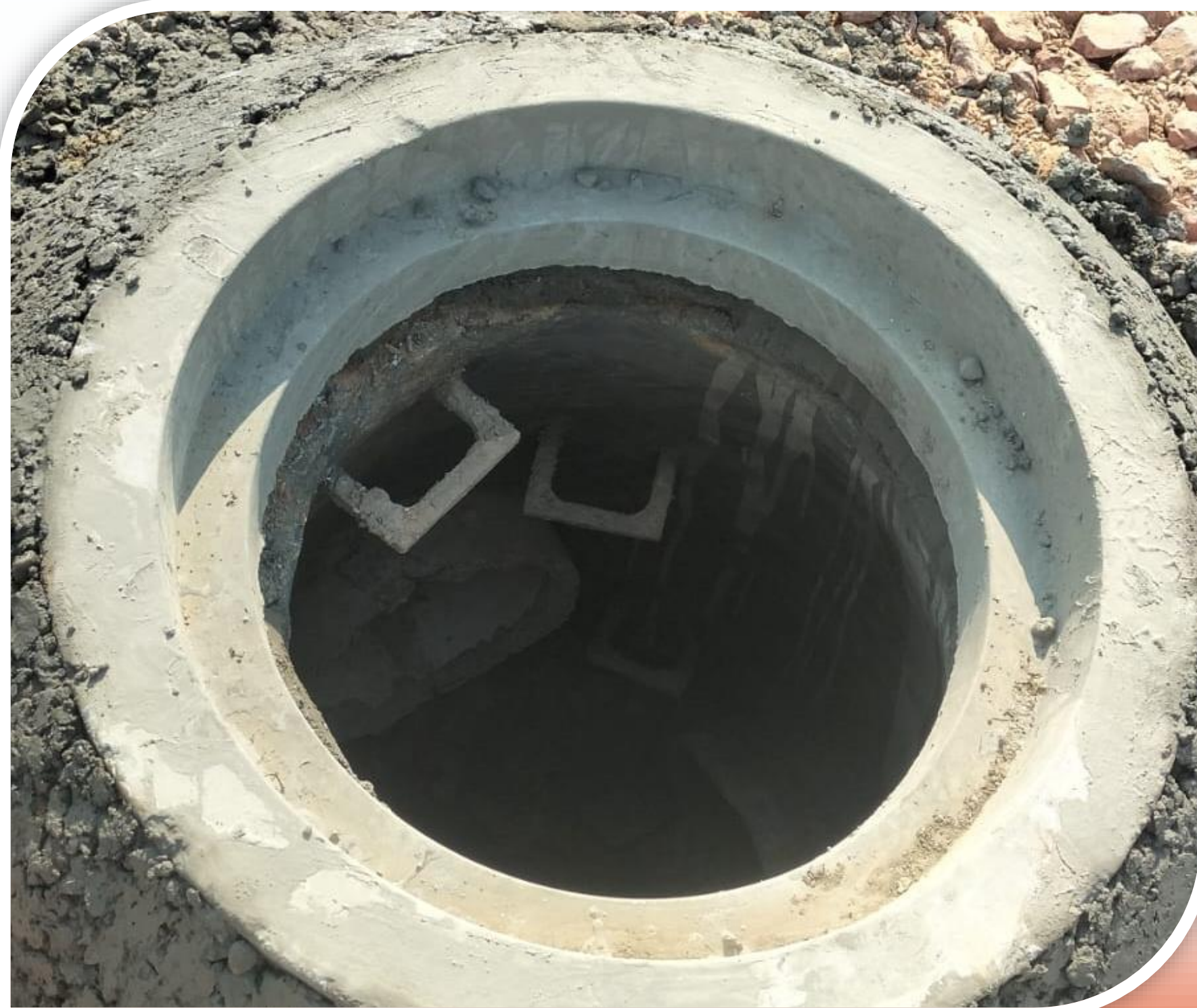
Sewer & Storm manholes completed
