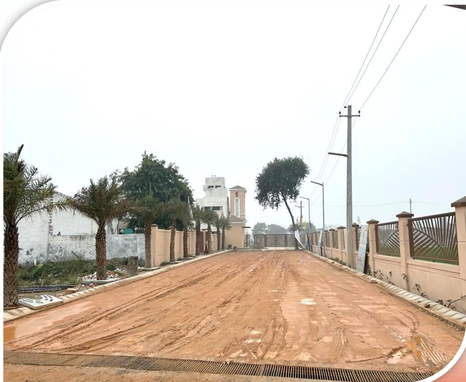
Road of entrance plaza ready for blacktop
