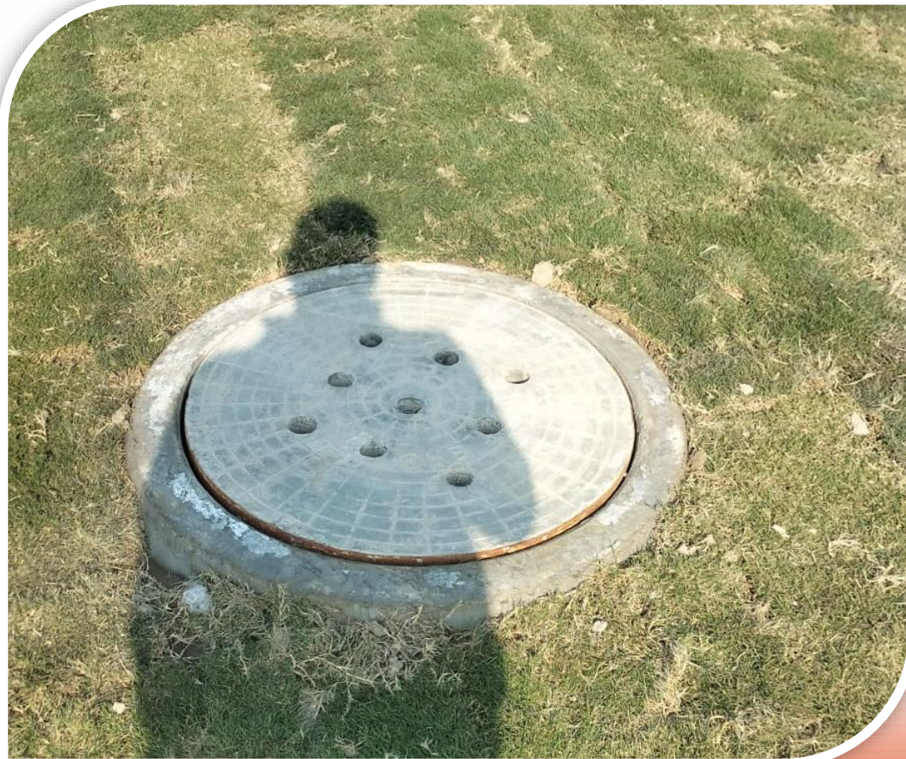
RAINWATER HARVESTING work completed
