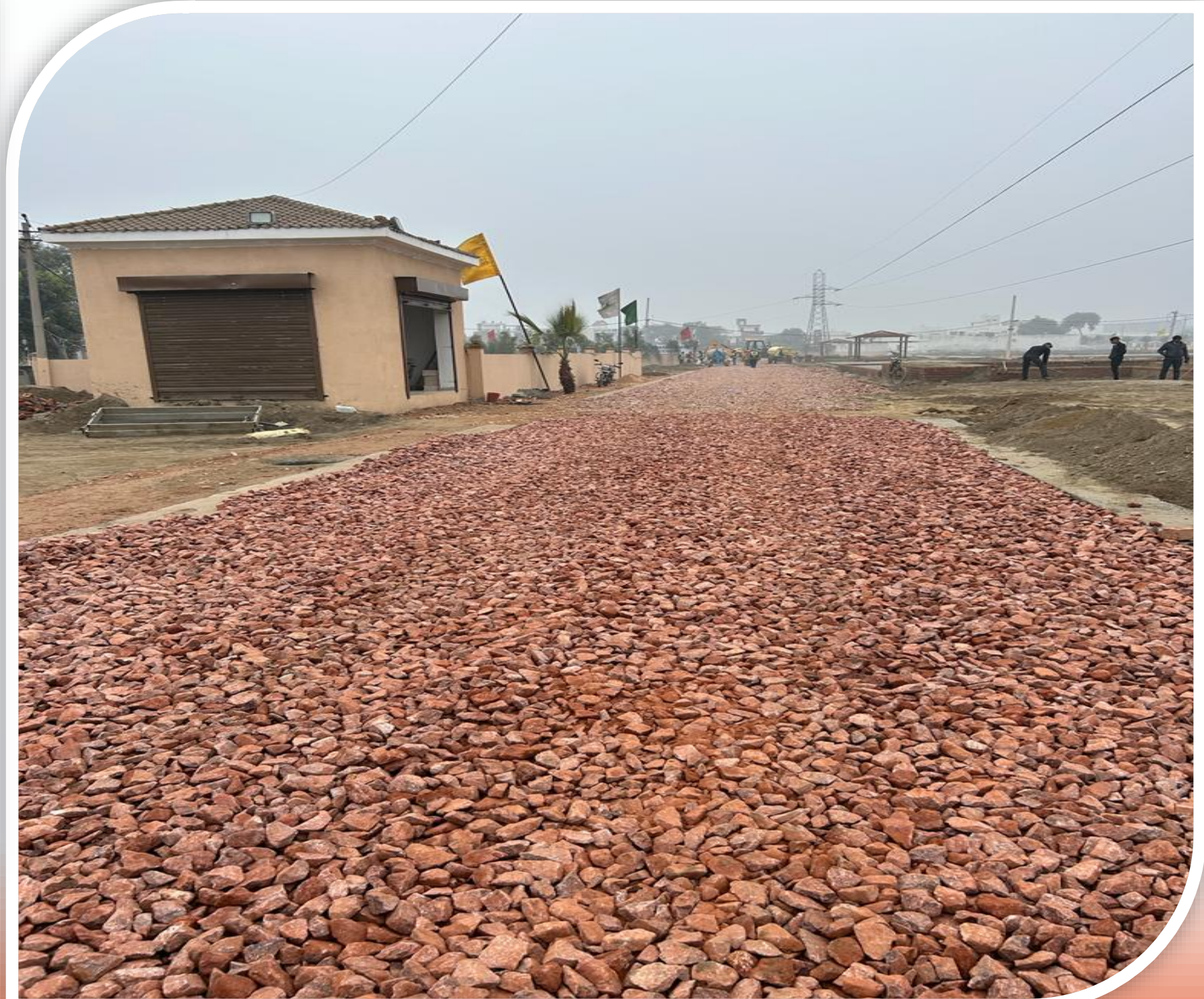
Road final sub-base work in progress
