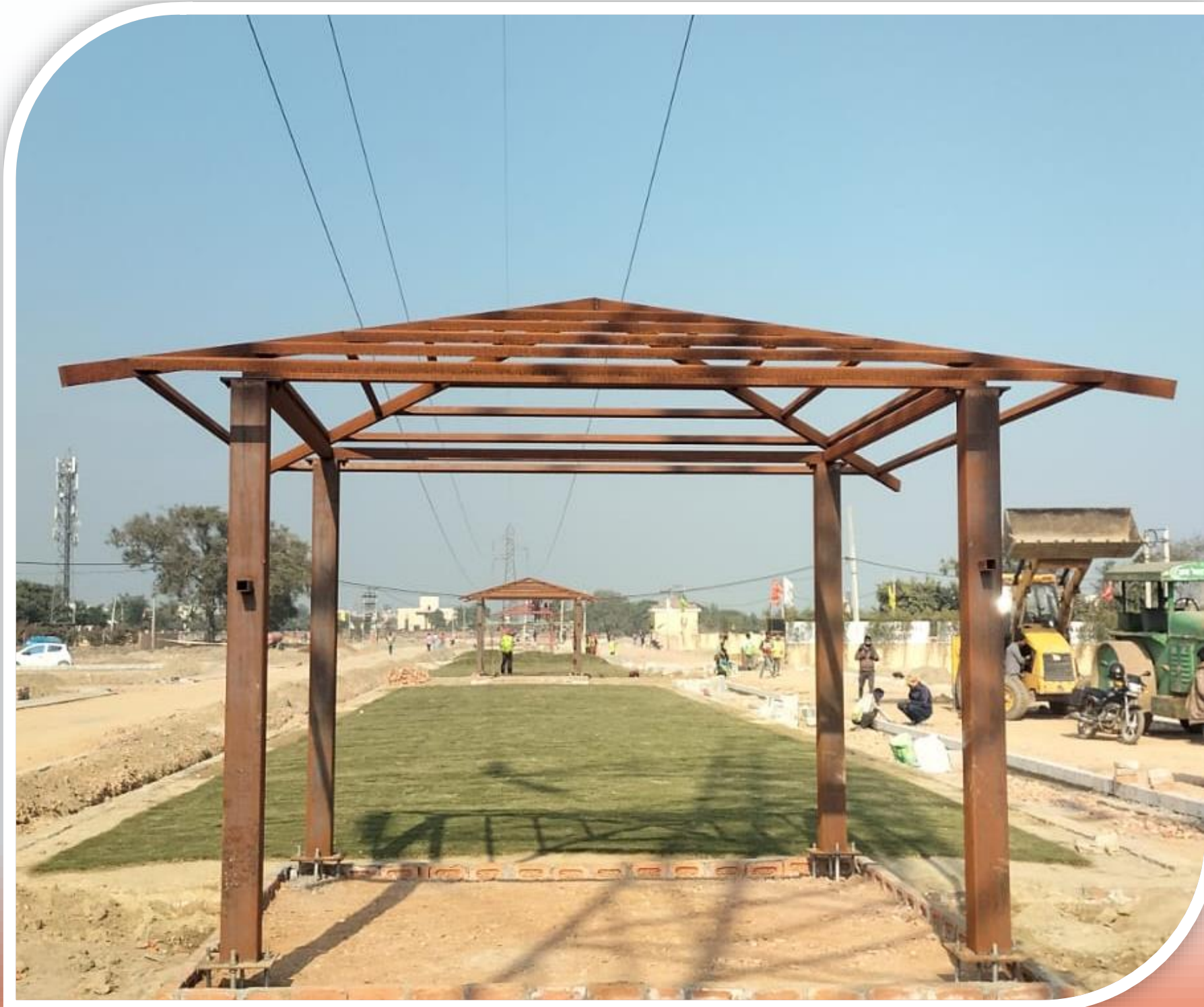
GAZEBO & civil work completed
