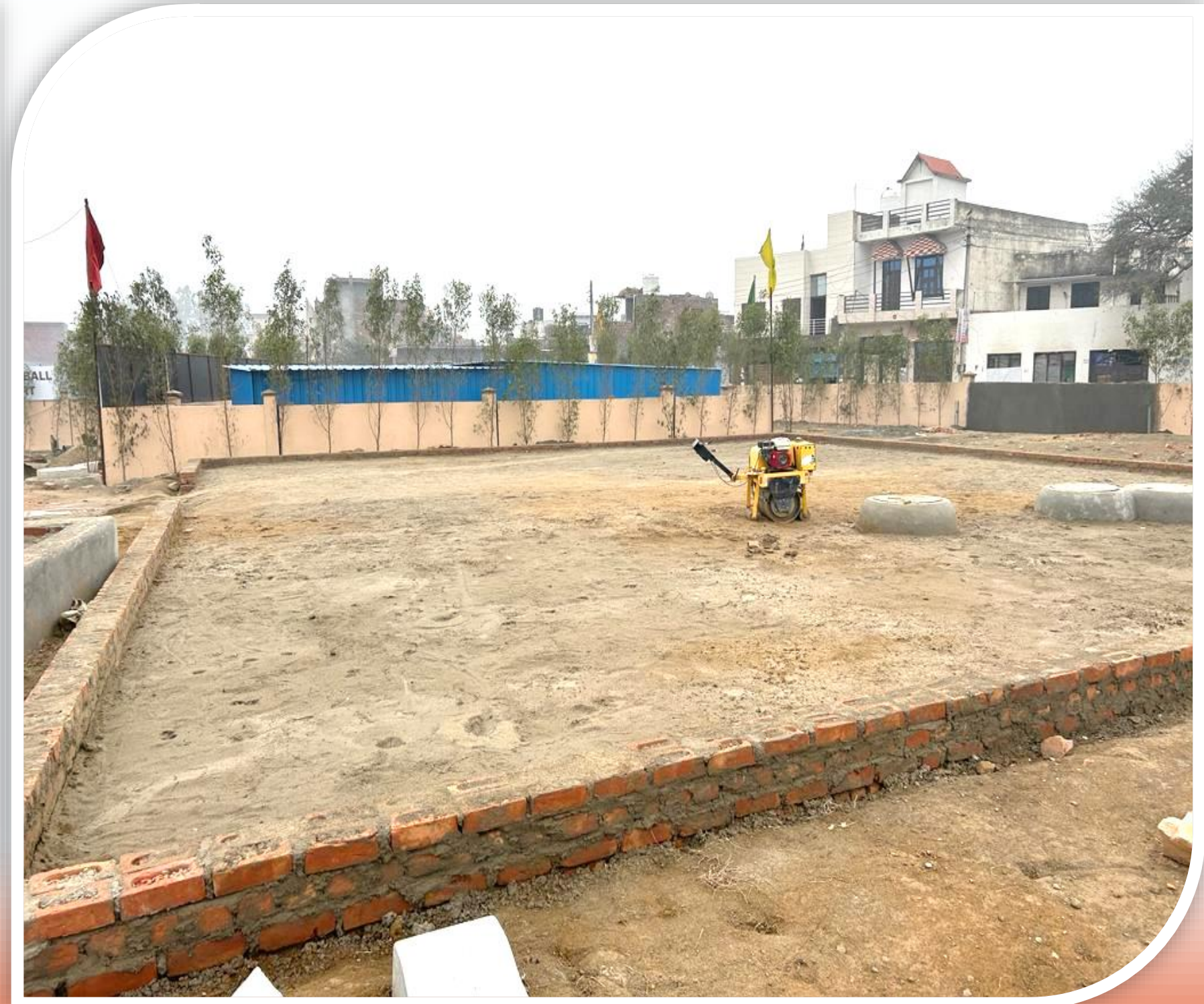
BASKETBALL civil work in progress
