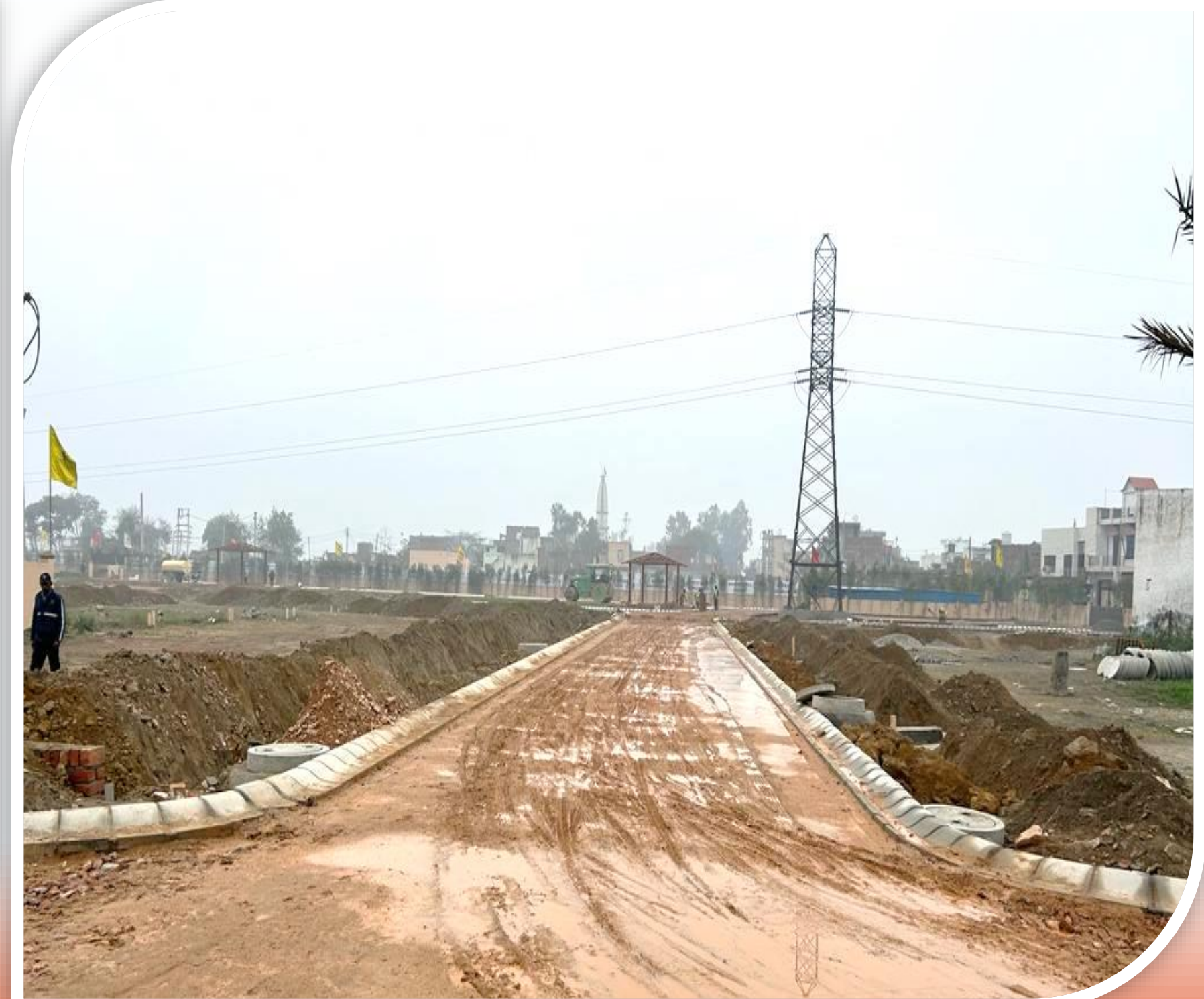
Kerb stones installed & ready for blacktop
