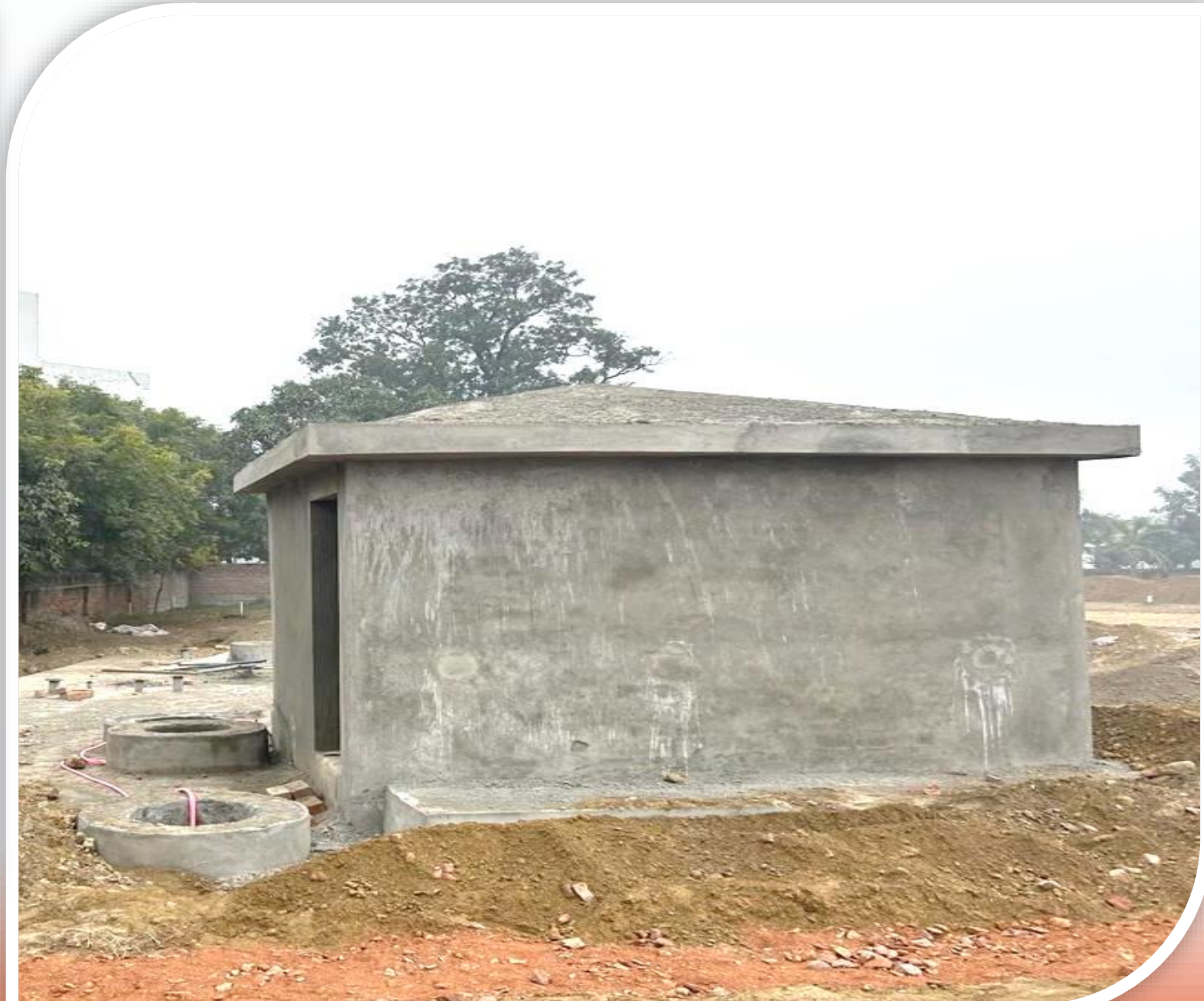
UGWT structure completed
