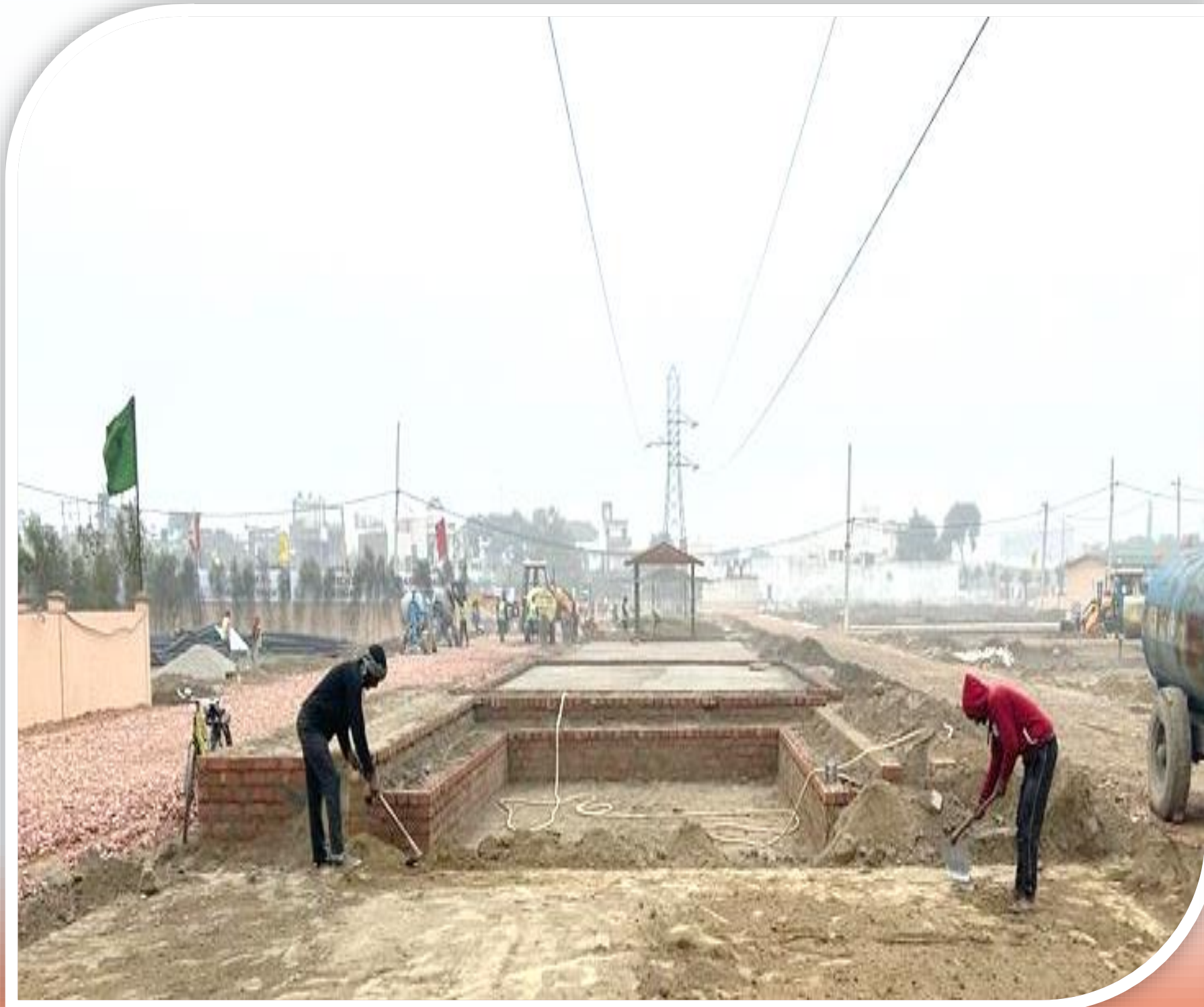
OAT civil work completed
