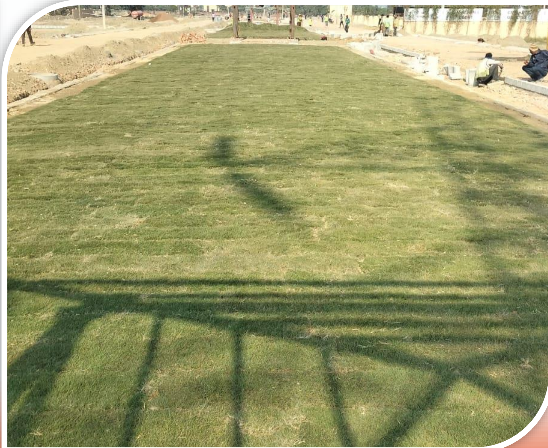
Park structural & grass work completed
