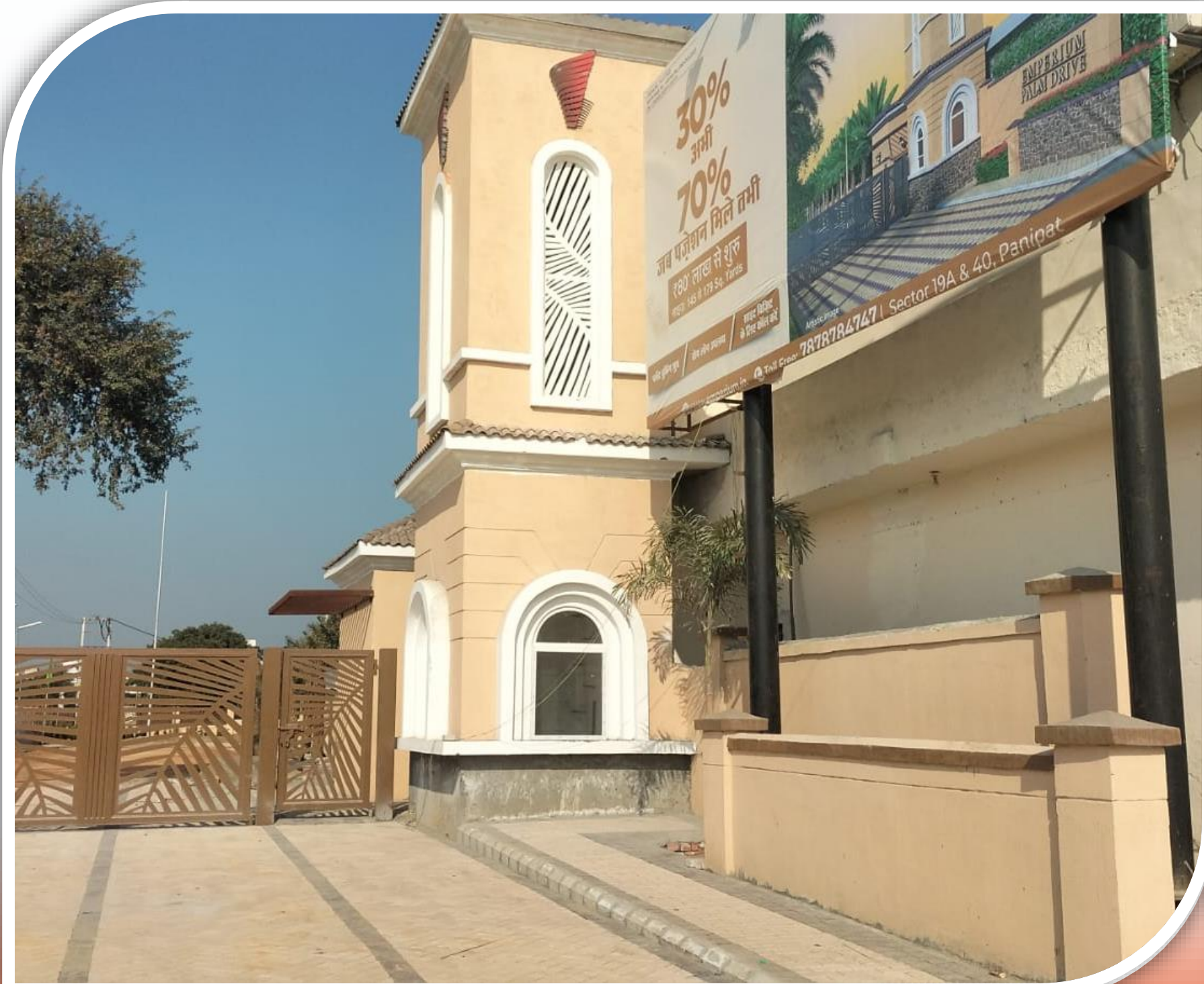
Guard room completed
